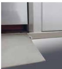
Insulating the bottom of the oven or fermentation cabinet saves substantial amounts of energy. It also prevents damage to floors and further improves fire safety.
